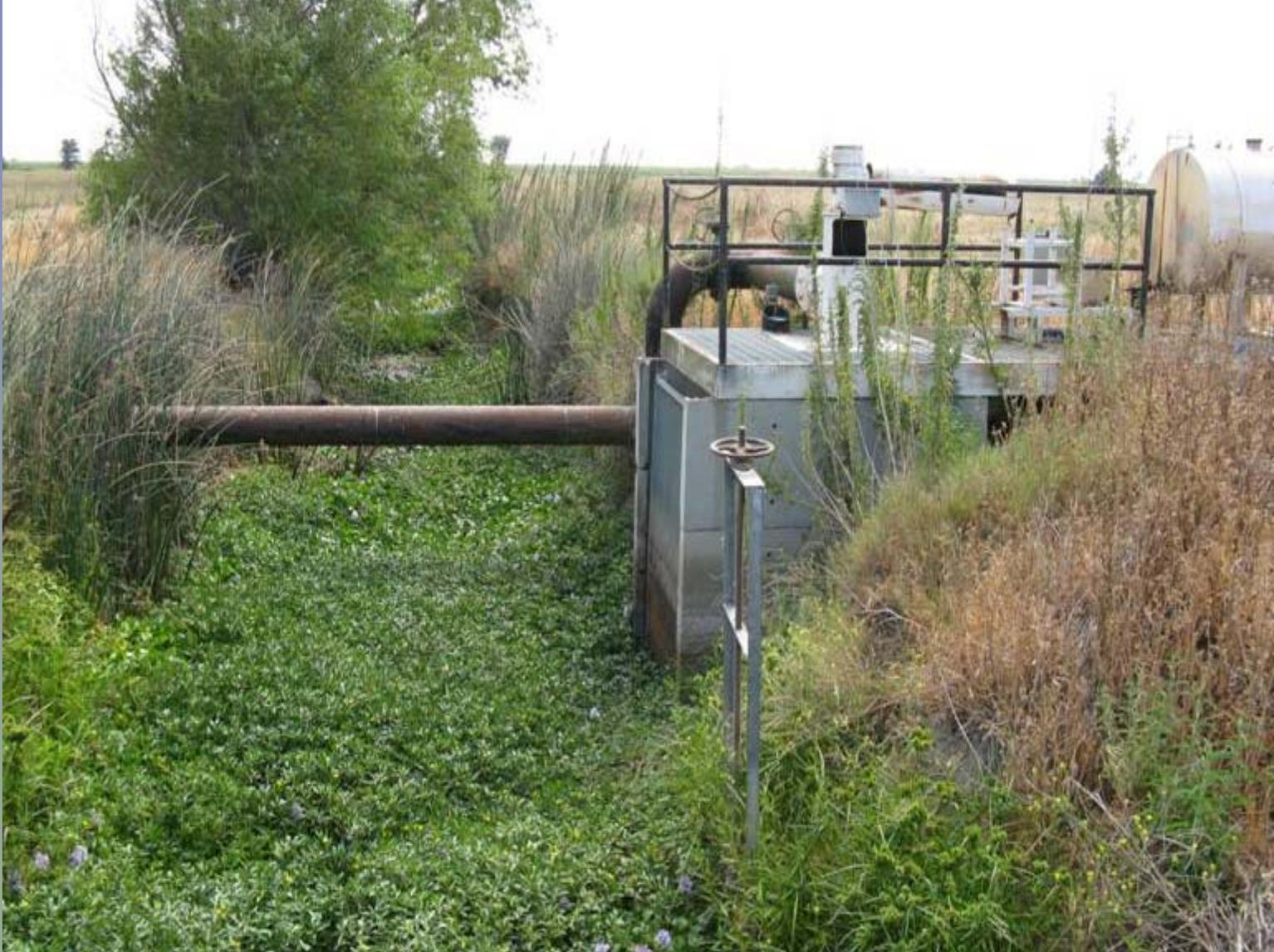
Existing lift pump at Woodbridge ER needs rehabilitation and new motor.
