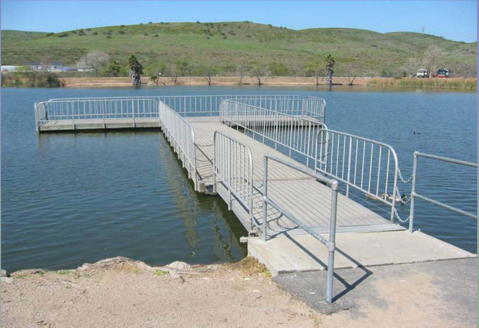
This is one of the two piers to be replaced; the vertical posts are supporting the end of the pier because the floats underneath have deteriorated.
