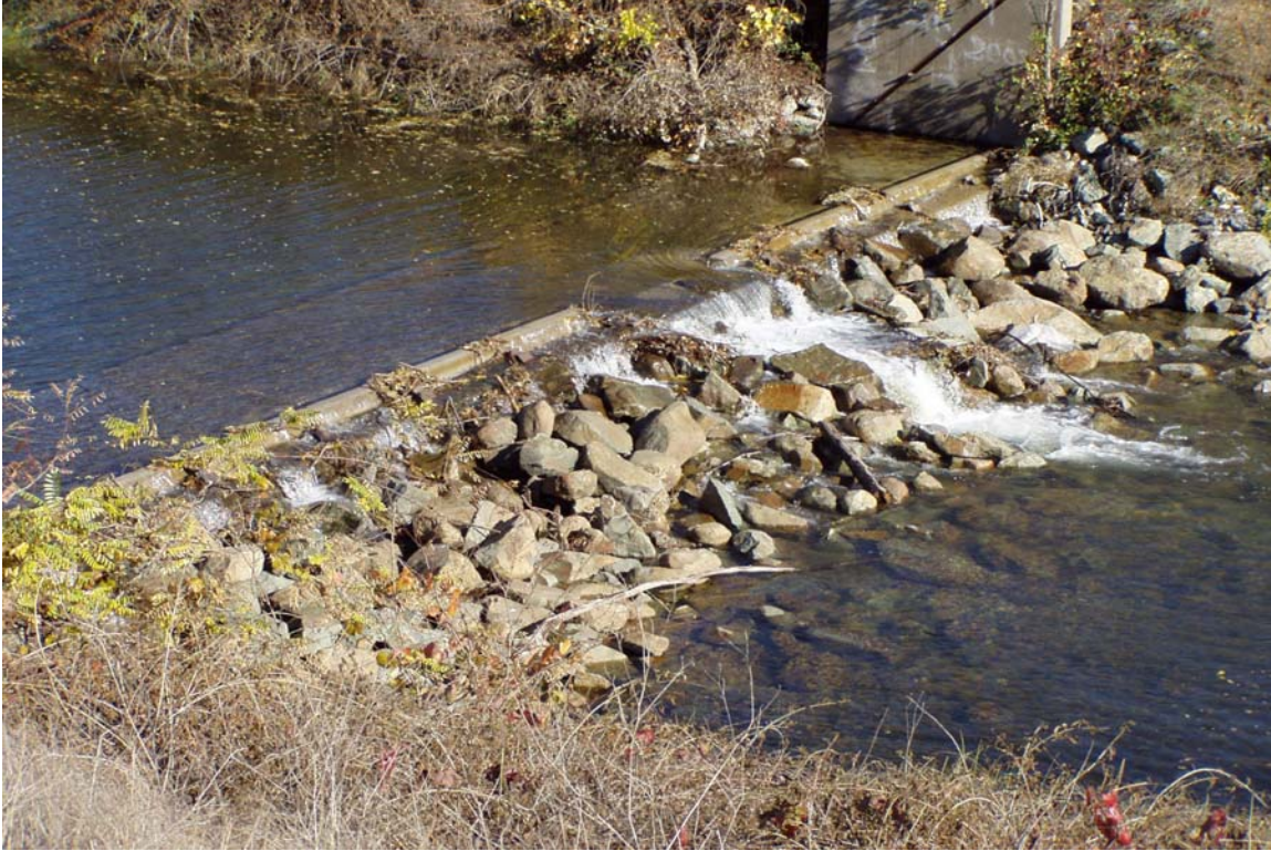
Figure 5 Rooney Dam following improvements made in the 2003. Note the concrete curb on the weir footing and the focused flows in the modified rip rap channel. The steep rock approach still remains problematic to upstream migrating salmon during flows less than 70 cfs.
