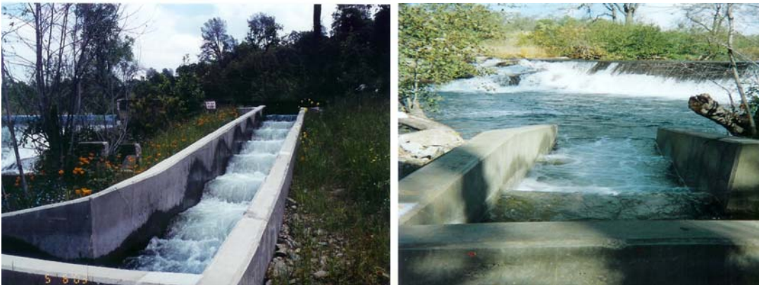
Figure 7. New ladder on South Granlees Dam. Photo on left shows upper section of new ladder with higher walls and reduced jump heights. Photo on right shows new outlet location away from false attraction flow.
