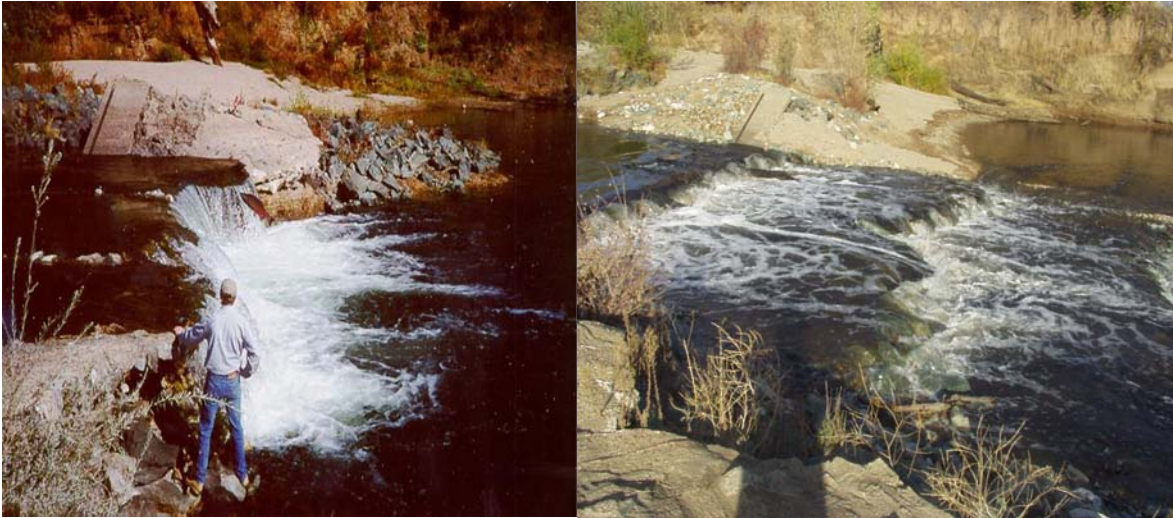
Figure 4. Blodgett Dam prior to (left) and following improvements(right). The photo on the left was taken during the stranding event. Note the salmon jumping in the center of the photo.
