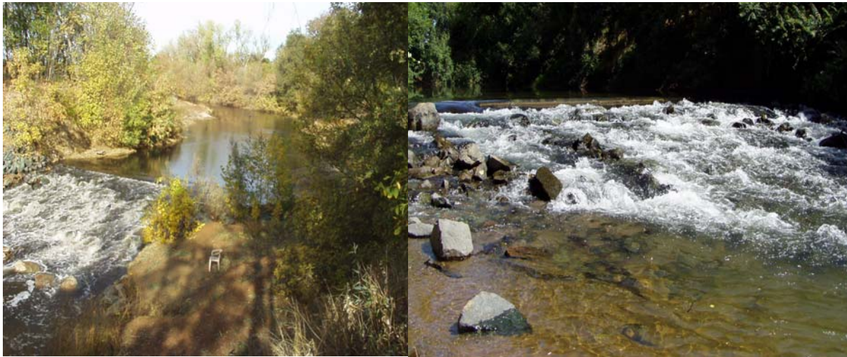
Figure 3. Hop Ranch (left) and Mahone Ranch (right) following improvements made in 2002 and 2003 respectively. Note the low angle rock approach on both structures.
