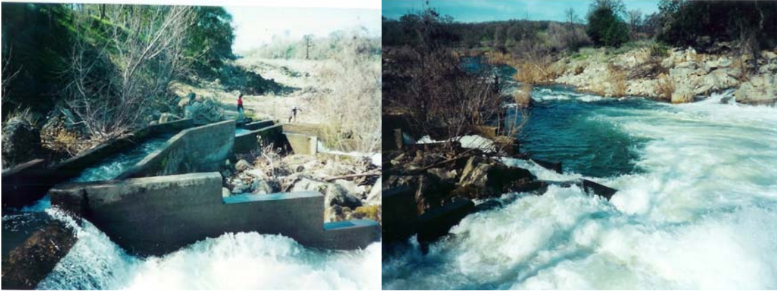
Figure 6. Granlees Dam fish ladder pre project. Photo on left shows short walls and turbulent flow in pools caused by inadequate volume. Photo on right shows the outlet of ladder adjacent to mis-directing attraction flow at dam face.
